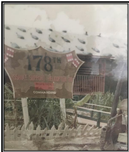
The 178th Assault Helicopter Company Headquarters in Chu Lai, Vietnam, 1971. Note the sandbags weighing down the roof of the hooch against the ravages of typhoons. Photo by Steve Wolak.
