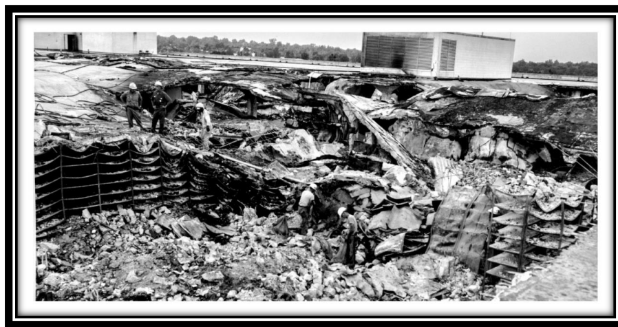
NPRC fire aftermath, July 1973. (Photo credit: National Archives)
